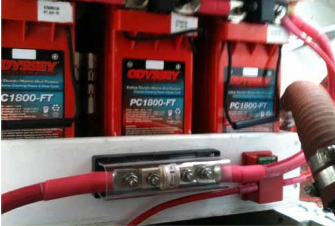
Battery bank complete, with wiring and fusing
